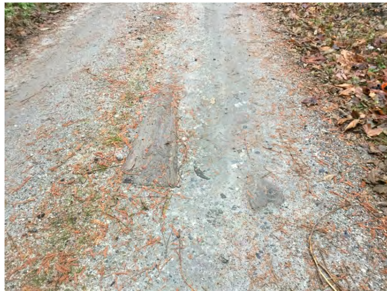
Top layer of stringers right at running surface
