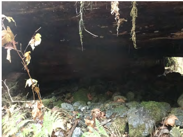
Left Bank Abutment when facing downstream
